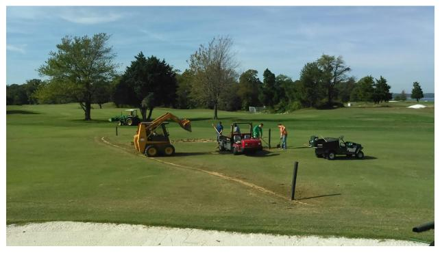
Figure 7. Drainage project on #18 fairway at Cedar Point Golf Course. Water is carried back and empties into an irrigation pond providing up to 1 million gallons of recovered rainwater each year. Photo credit: David Burkhart.
