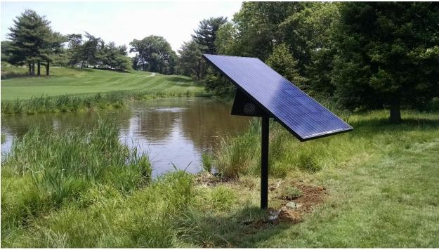
Figure 18. Artificial aeration helps to maintain DO levels, like this solar powered sub-surface aeration system in use at the Army Navy Country Club. Photo credit: Sandra Burton.
