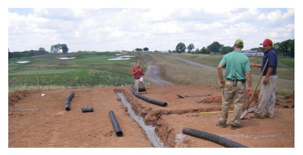
Figure 4. Drainage installation during the construction of a new tee. Photo credit: Thomas Turner.
