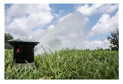
Figure 11. Irrigation heads can be brought on-line for a few seconds and observed for proper operation. Photo credit: Mark Jones.
